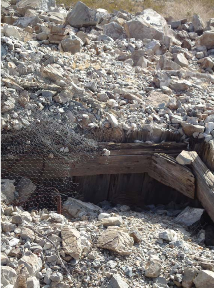
Figure 5: One of about a dozen historic old shafts seen around the property, which now are routinely filled as a safety precaution
