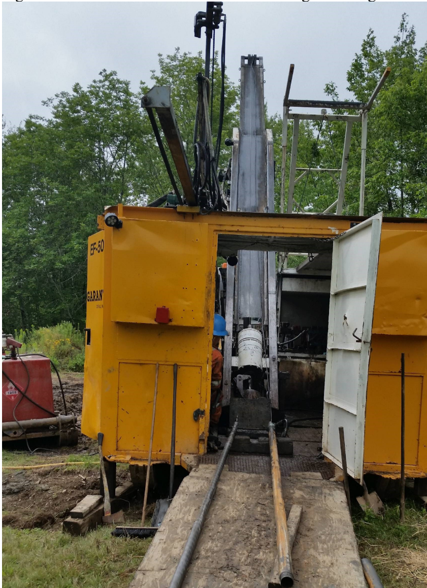
Figure 3: One of Two Diamond Core Drill Rigs Running
