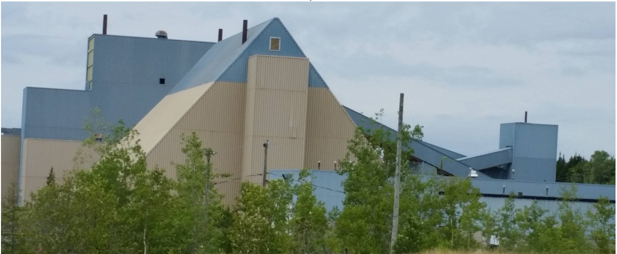
Figure 7: Mt. Pleasant standing mill processed 990,000 tonnes of tungsten ore in 1983-84; ball mill removed but remainder of infrastructure, froth floatation cells and tanks remain
